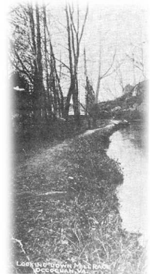
THE OCCOQUAN - The water holding tanks now occupy this spot shown at the turn of the mill race.
